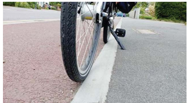
An example of a 'forgiving kerb': a gentle slope allows cyclists to join or leave the track where they like
