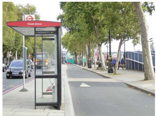
Unlike the above example, this cycle highway offers access to the footway via dropped kerbs and raised tables
